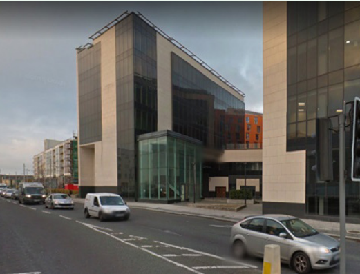
The Simms Building
